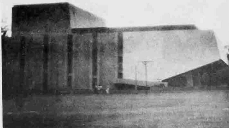
CULTURAL SEAT — Dumaguete is earning a name as the South's cultural seat with the construction of the Luce auditorium at the Silliman University.
