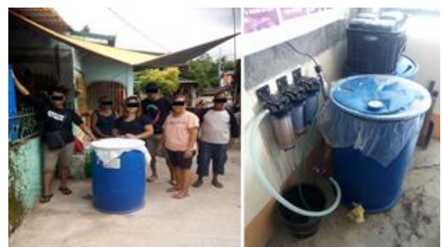
Figure 13: Improvised rainwater collection using tarpaulin and drum
